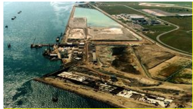
Fig. 6 Tunnel of the Øresund Bridge [22]
