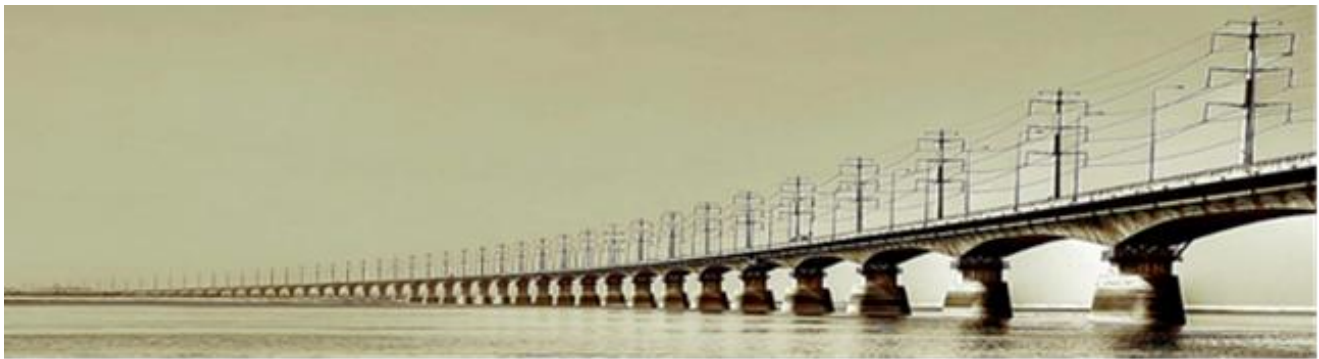
Fig. 7 The Bangabandhu Jamuna Bridge [27]
