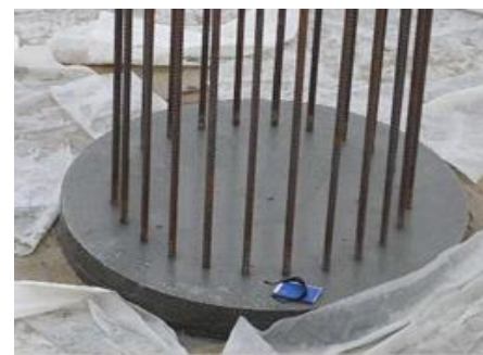
Fig. 19 Pile Head Waterproofing System
