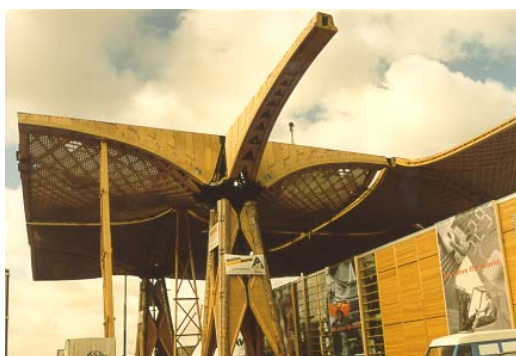
Figure 4.4.4: The leg and large girders are assembled from two box-beams. The length of the girder is 18.6 m.
