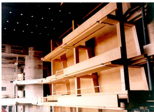
Figure 4.4.2: Sibelius Hall, in Lahti, Finland, used PU gluing with screw pressing technique in balcony elements, wall structures and ceiling elements.
