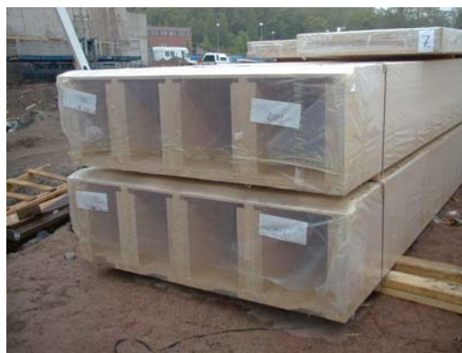
Figure 4.4.3: LVL stressed skin panels as balcony elements stored in the construction site.
